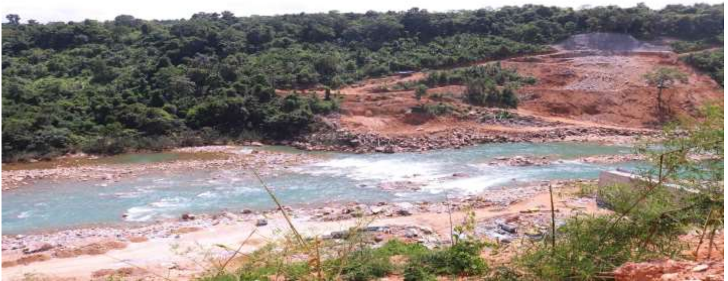
Pic: Dam site of Lower Kopili Dam in Assam
