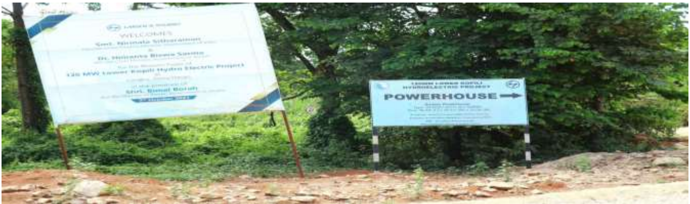
Pic: Power House Site of Lower Kopili Dam
