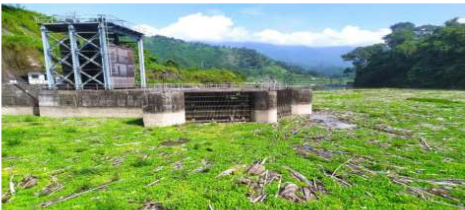
Pic: Reservoir of Pare Hydroelectric Project submerging agriculture land and forest areas.
