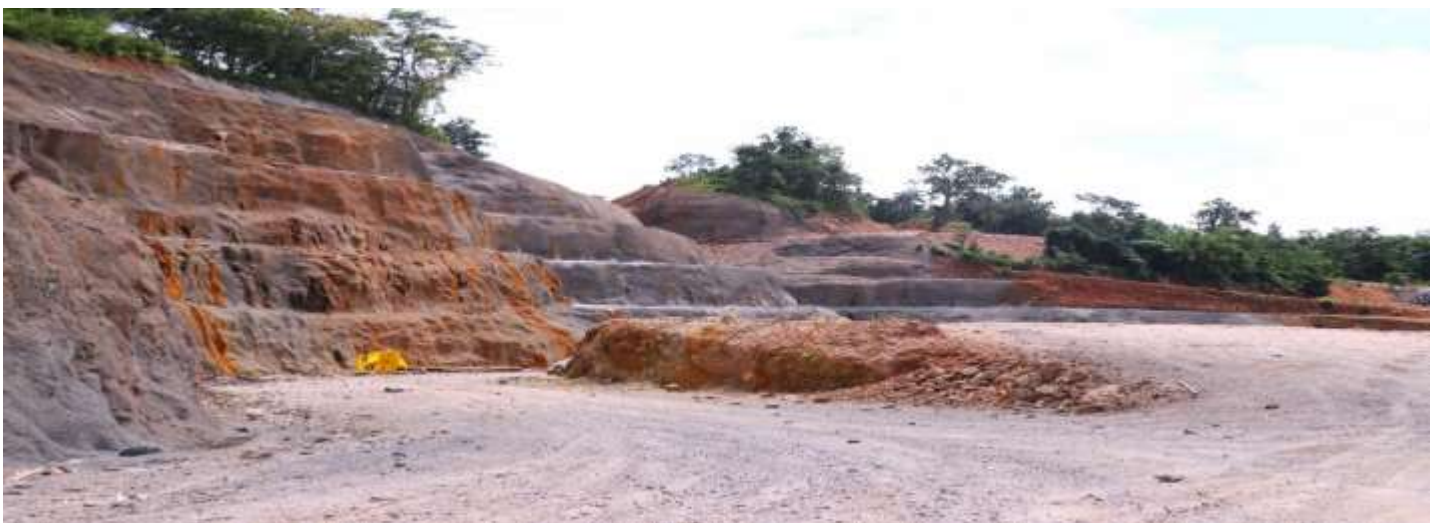
Pic: Site of Power House of Lower Kopili dam
